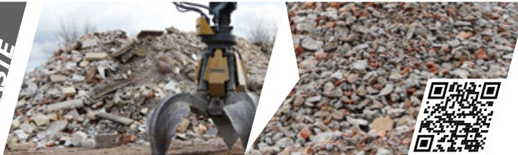
Mixed construction waste contains both, mineral (stone, brick, concrete) and non-mineral components (metal, wood, glass). In short: everything that is left behind during demolition. The raw materials produced after crushing are returned to the economic cycle as secondary raw materials.
